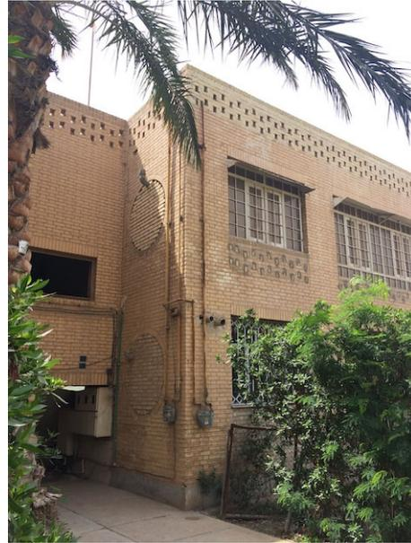
Figures 34 and 35: The recent state of circular openings in separating walls and balconies: (left) one of the few surviving openings in its original form; (right) balcony openings that have been completely covered with brick. (Photo credit: the author; 2018)
