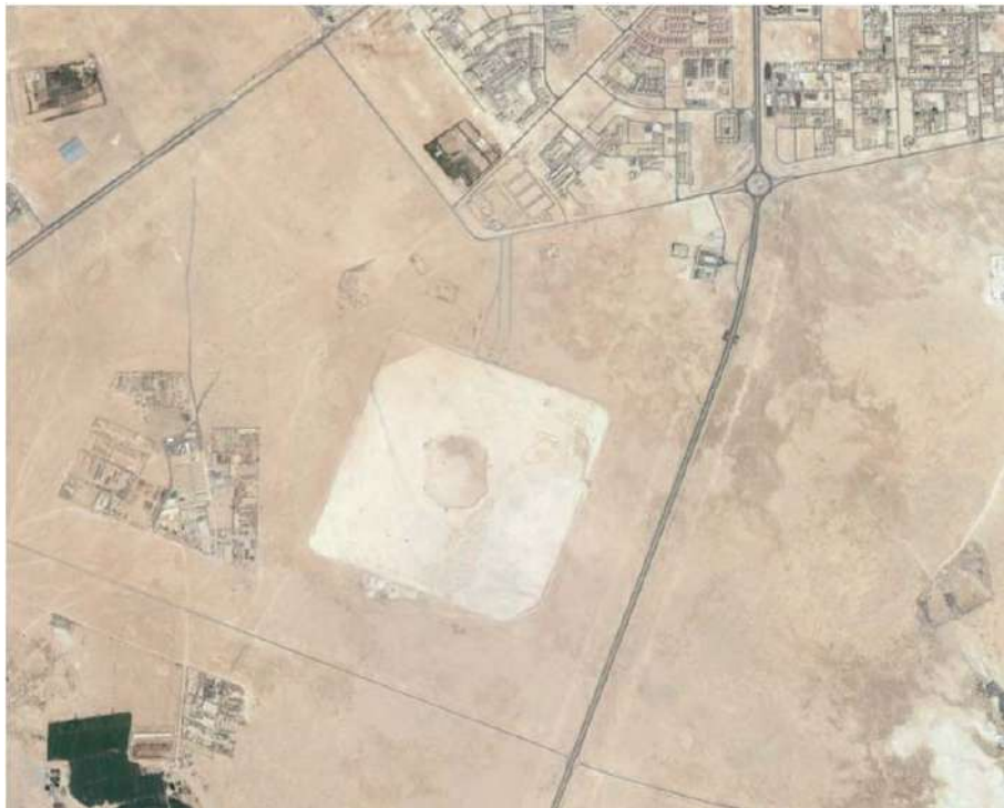
Figure 6. Aerial view of Al Khor stadium (Adapted from Google Earth).
