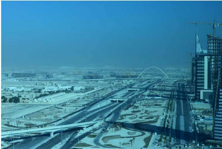
Figure 4. The area of Lusail under construction.
