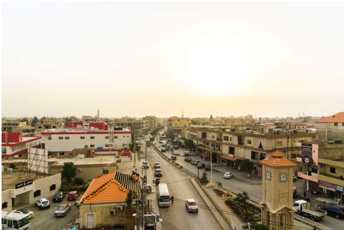
Figure 24. Bar Elias entrance road, Bar Elias, 2018
