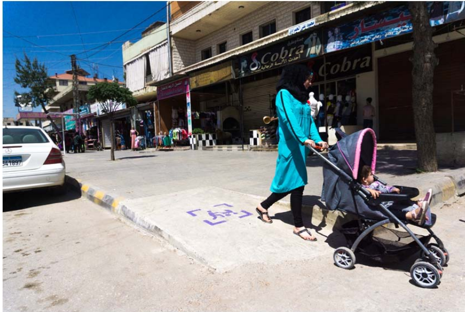
Figure 28. Access ramps created along all the sidewalks, Bar Elias, 2019
