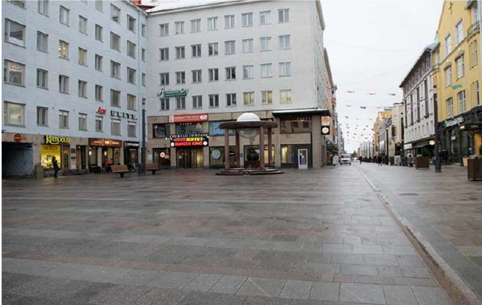
Figure 3. The heated pavement of the pedestrian street keeps the walking conditions similar all year round. The surface eases walkers and strollers to access the street in all weather conditions yet it is aesthetically poor (Oulu). (Source: Essi Oikarinen)
