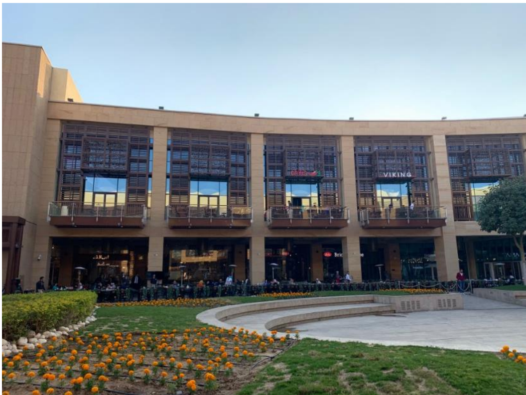
Figure 10. Wood screens combined with panes of coloured glass shade the façades that overlook the open-air plaza with landscaped garden, seating areas, and water feature. (Source: Foursquare City Guide – User Photo)
