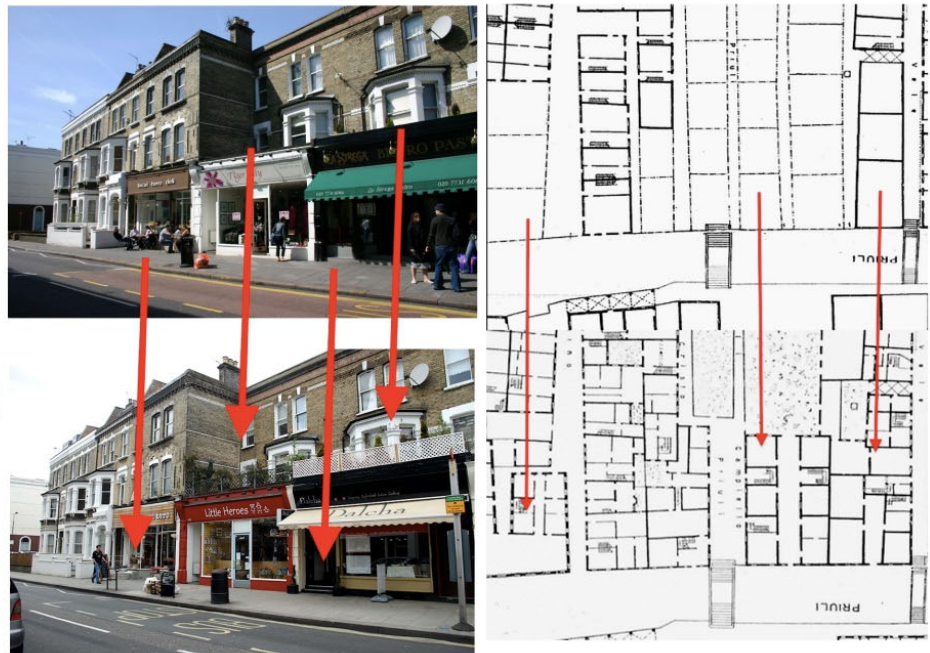
Figure 4. We are constantly co-producing and transforming our room-like public as well as private spaces, our “place networks,” over many scales of time. We open windows, close doors, remodel spaces, and make longer-scale transformations, like the changes over five years in London (centre) and over a century in Venice (right).
