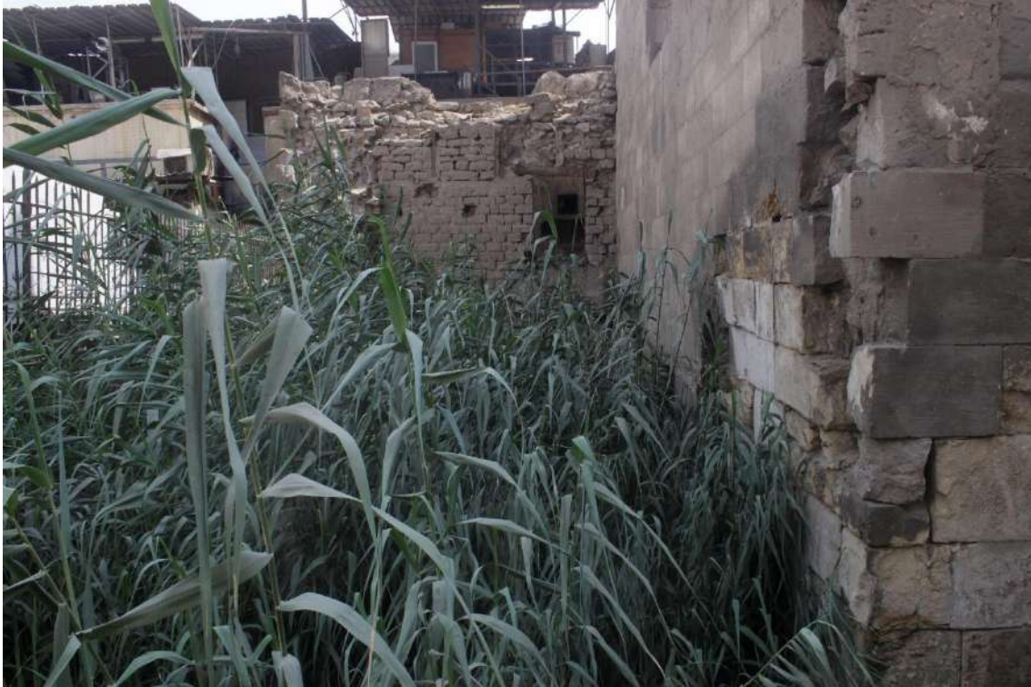
Figure 9. Groundwater damage at al-Ashraf Khalil Dome in al-Khalifa Street © Athar Lina
