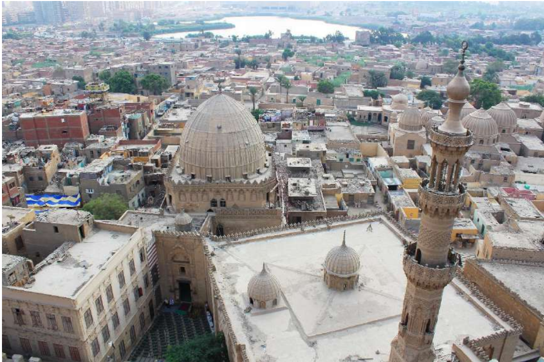
Figure 15. Al-Imam al-Shafi' Mausoleum with al-Shafi'i cemetery and 'Ayn al-Sira Park in the background © Athar Lina
