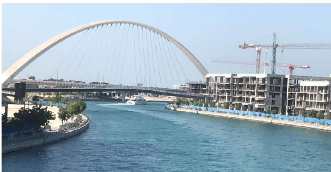
Figure 7, 8, 9: Prominent features across Water Canal (Source: Author's Photograph)
