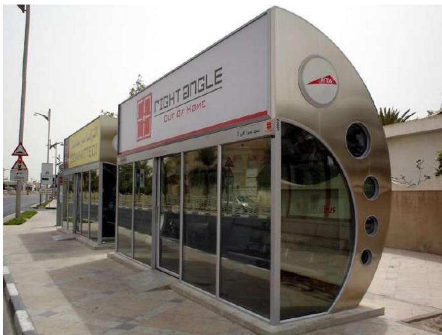
Figure 13. Air-conditioned bus shelters in Dubai – retrieved from www.arabianbusiness.com
