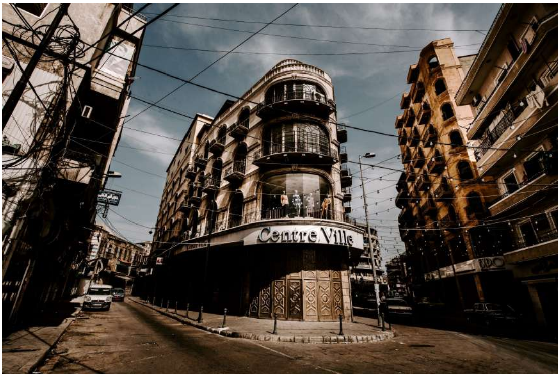
Figure 2. Buildings in the Old Tripoli downtown, al-Tall Square, built during the French colonial time. Photo credits: Malek Haddad.
