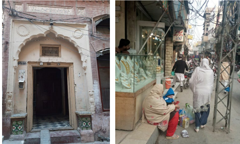
Figure 13 (left). Built-in benches with entrance of historical houses (Source: Authors) Figure 14 (right). Customers resting on a shop step called thara, in the absence of sitting spaces (Source: Authors)
