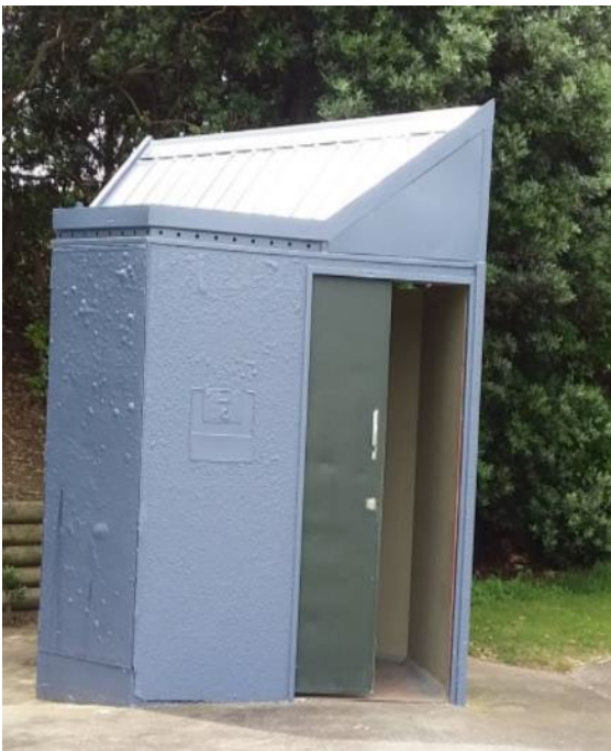
Figure 2. Existing toilet at Te Pua Keith Park.
