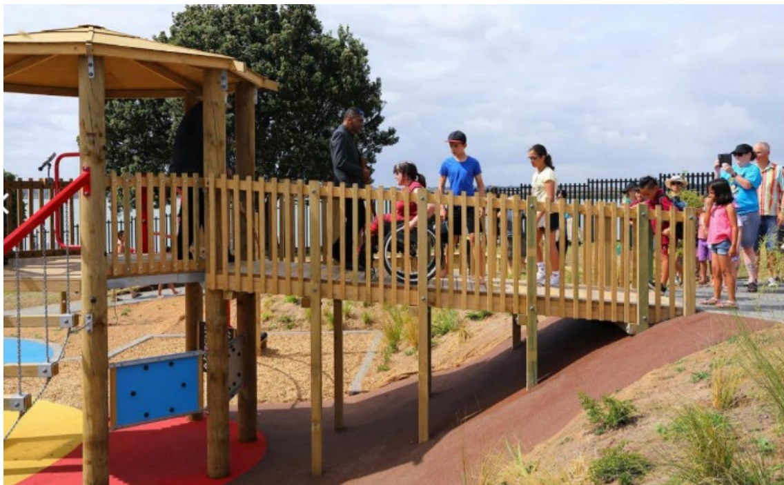
Figure 13. Gentle gradient ramp to the play tower.
