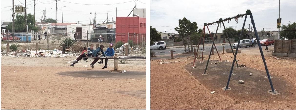
Figures 19 – 20. The condition of the playing equipment and the park [source: author].
