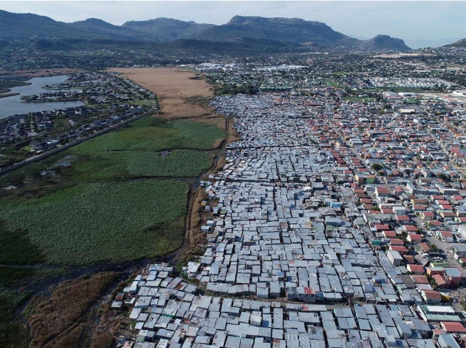
Figure 2: Wetland encroachment in Kommetjie. Source: Bruce Sutherland, City of Cape Town.
