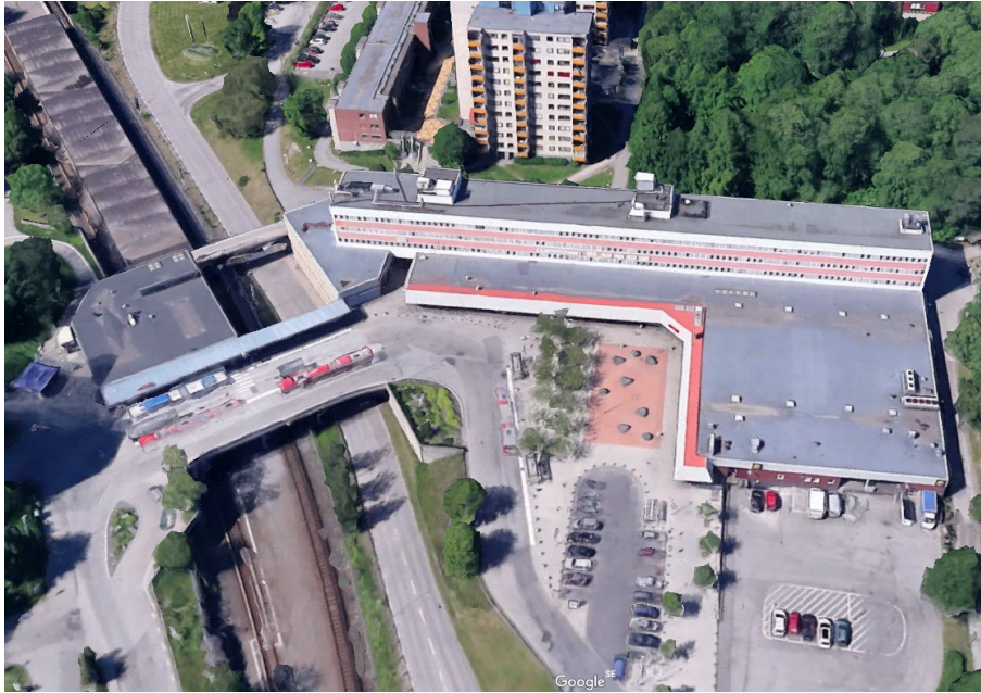
Figure 2. Overview of Fittja main square from. Source: Google Earth, 2019
