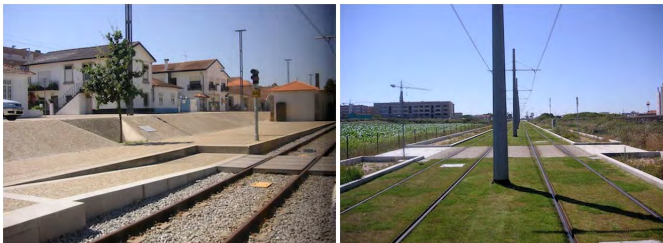
Fig. 5-6. Metro do Porto interventions in Maia (Eduardo Souto de Moura and João Álvaro Rocha) and Vila do Conde (Eduardo Souto de Moura and José Gigante). Source: author.
