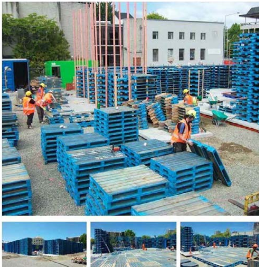
Figure 3: Pallet Pavilion during construction 2012.
