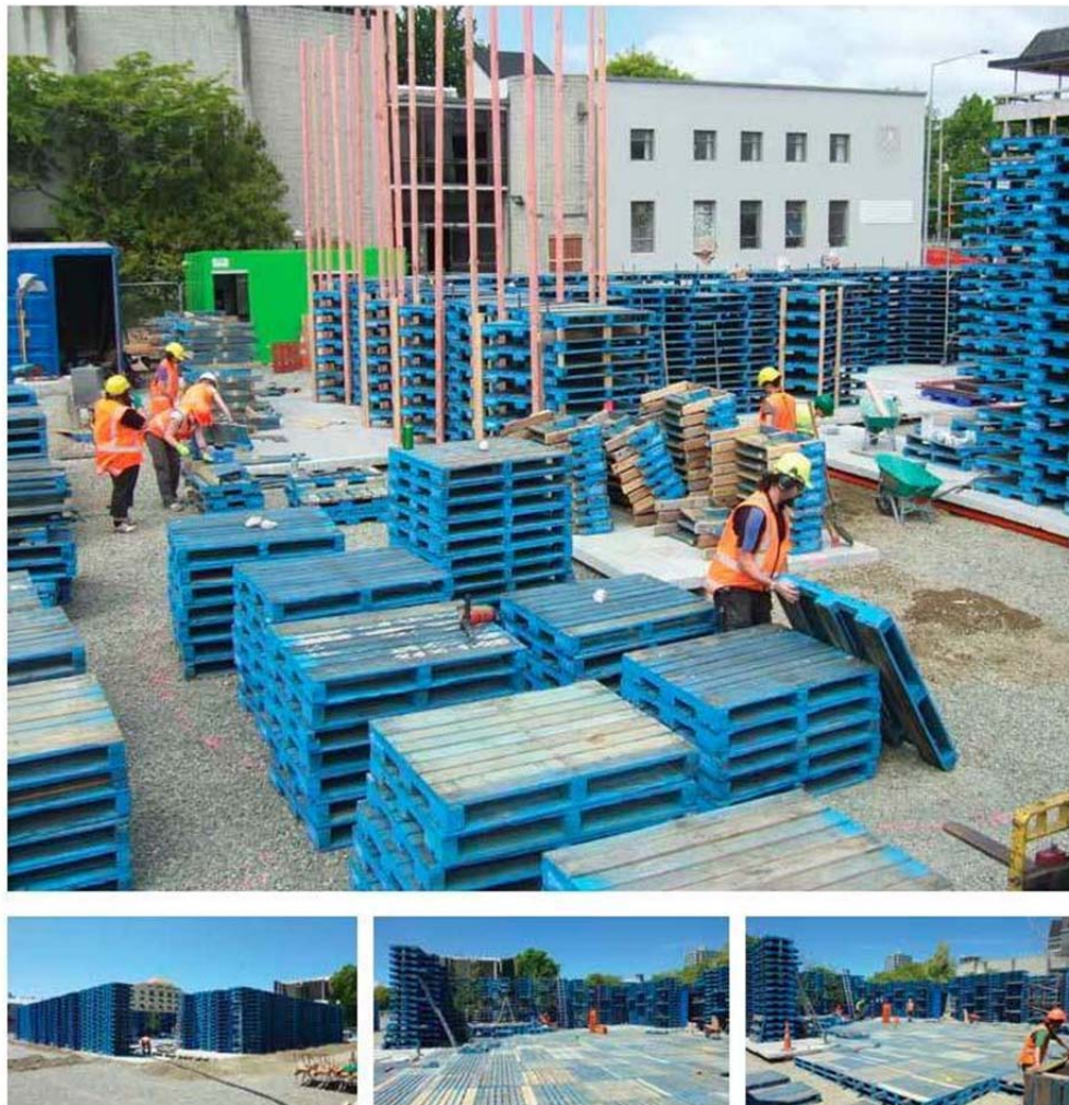
Figure 3: Pallet Pavilion during construction 2012.
