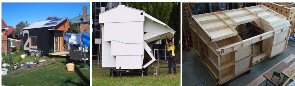
Figure 1. A selection of projects from the LBM digital fabrication research activity (left to right): The Castle2 in backyard setting; The Castle5 – unfolding; Scout-hut prototype).
