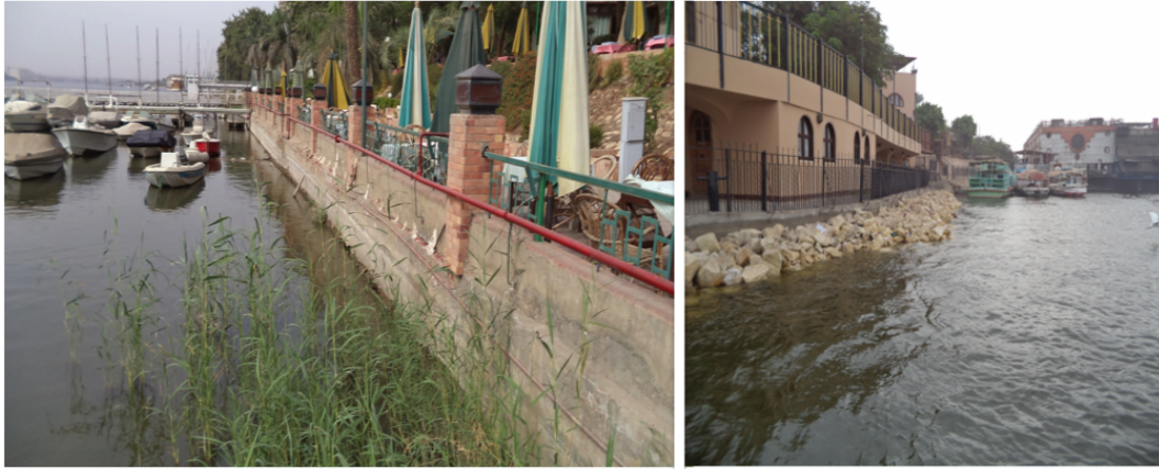
Fig. 22. Example of river edge with highly urbanized concrete banks (to the left al-Yacht club looking north and to the right al-Adra church looking south).
