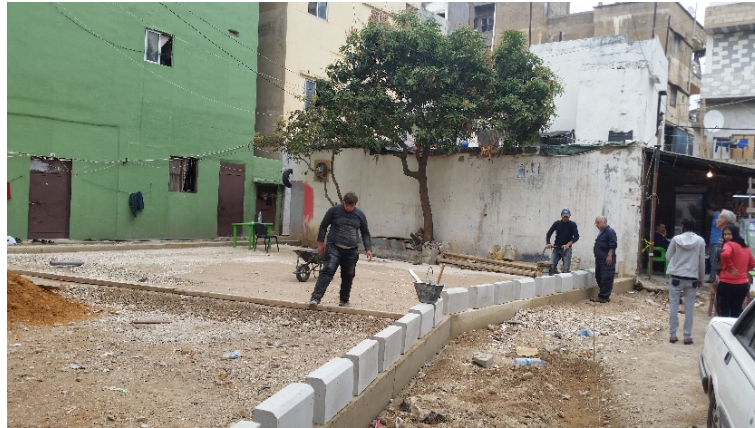
Fig. 24. Preparation of the pavement. March 2017
