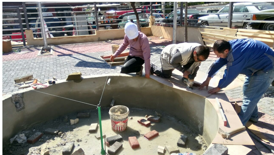
Fig. 14. The new fountain was constructed out of recycled materials from the walls of the old fountain
