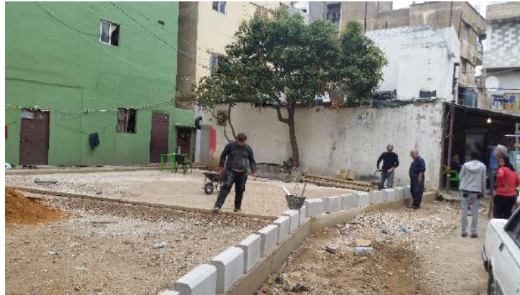
Fig. 24. Preparation of the pavement. March 2017
